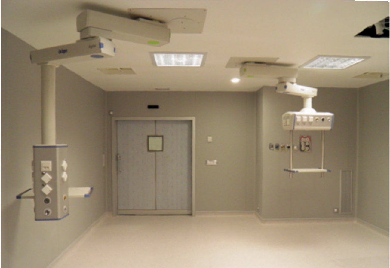
Hospital in Madrid, Spain
